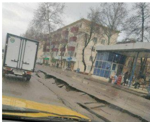
Figure 1. Automobile road collapse, Landslide of soil near the apartment building in Pakhtakor
