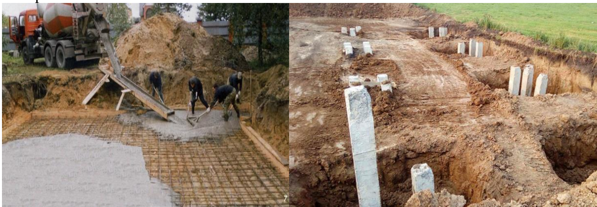
Figure 3. The basis of buildings and structures in saline areas increase durability
